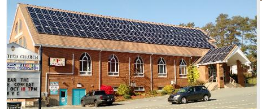
From start-up to completion
